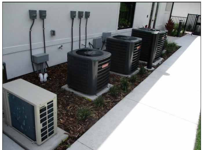
36. Pad-mounted HVAC split system condensers
