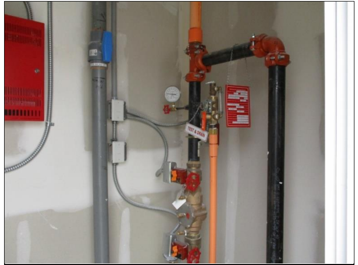
38. Fire sprinkler riser pipe at each building
