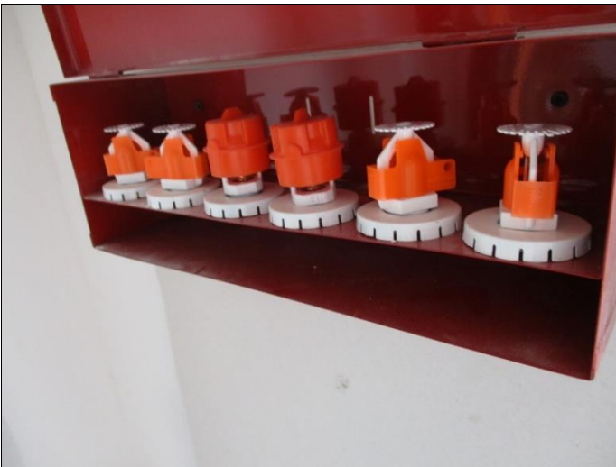
39. Replacement fire sprinkler heads
