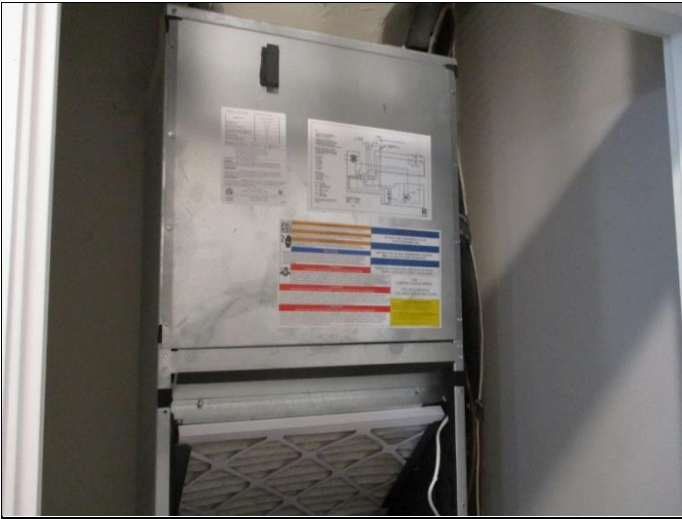
37. Split system air handler unit in mechanical closets in each unit
