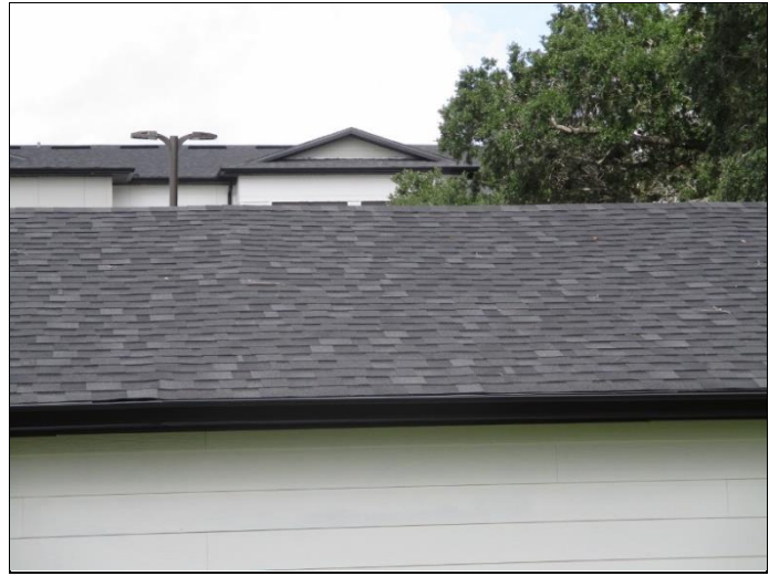
26. Pitched asphalt composite shingle roof finishes
