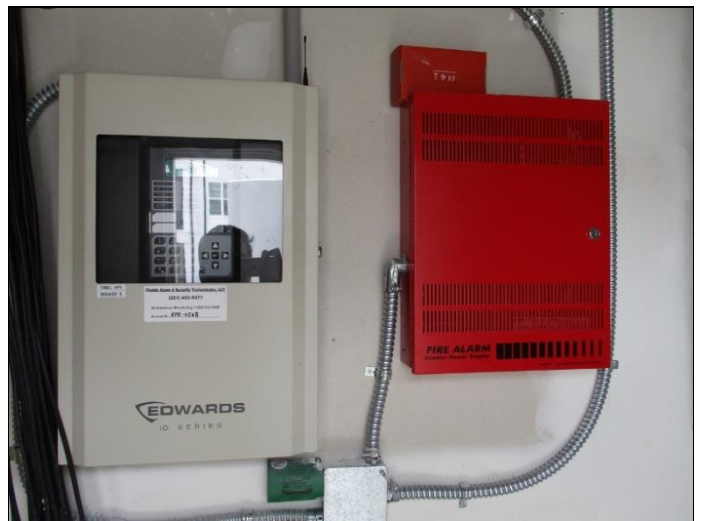
42. Central fire alarm control panel
