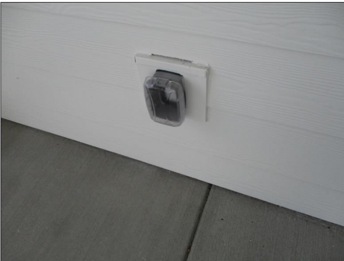
33. Exterior GFCI receptacles inside appropriate housings
