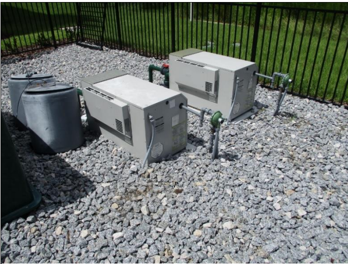
21. Gas-fired pool heaters
