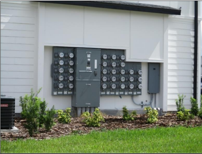
31. Façade-mounted electrical meters
