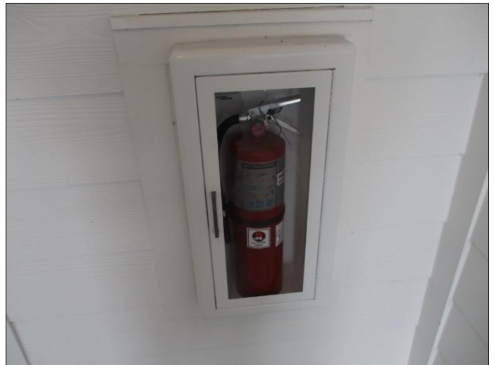
40. Fire extinguishers in mounted enclosures
